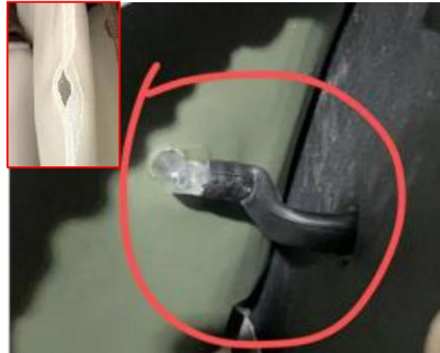
air hose folded and air bags broken
