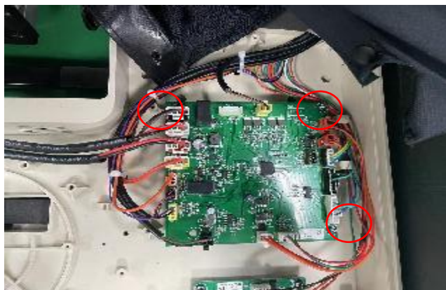
D.discontent the terminals and screws
