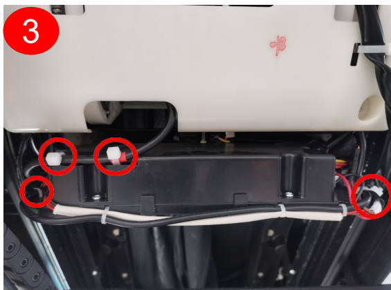
cut cable tie
