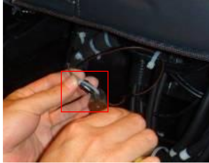
Cable ties tightening the wire and connector
