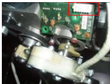
1 terminals on the board
