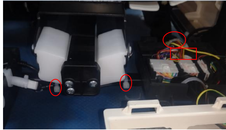
B.cut cable tie , disconnect the terminal
