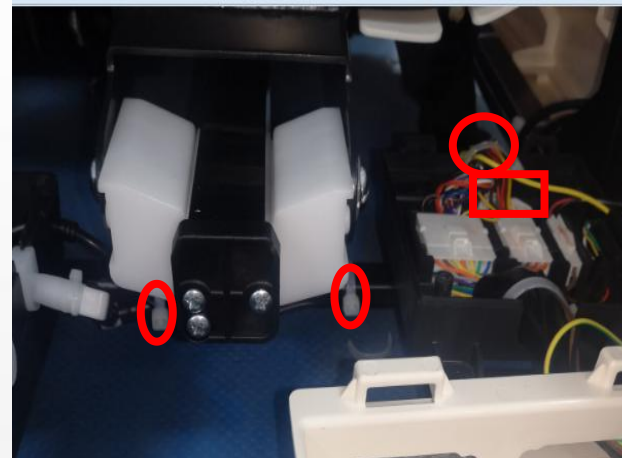
cut the cable tie and discontnet the terminal and air hose
