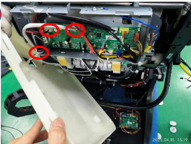
discontent the terminals and cut the cable tie
