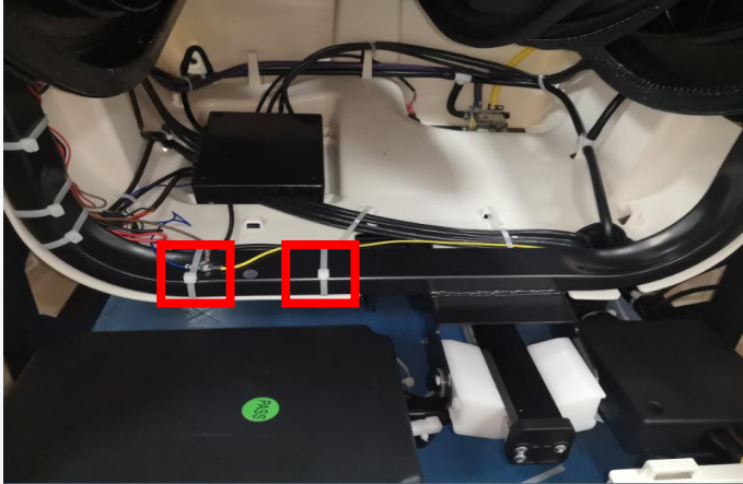
cut the cable tie
