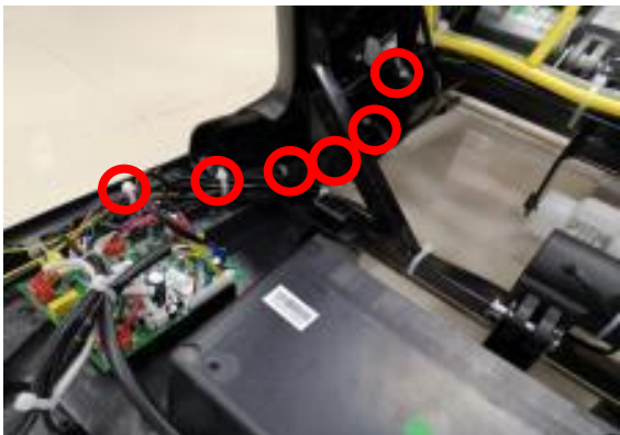
cut the cable tie
