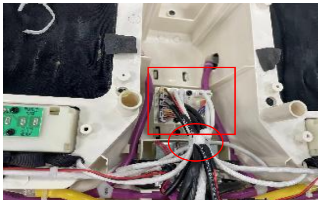
G.cut cable tie, disconten the terminals
