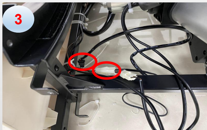
d. disconnected the terminals
