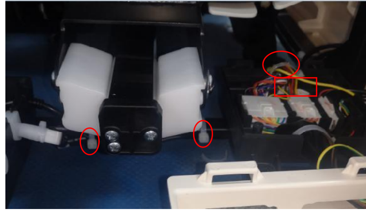
B.cut cable tie, disconnect the terminal
