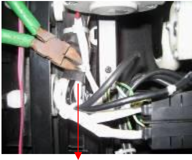
Cut the cable ties and remove close-end wire connector
